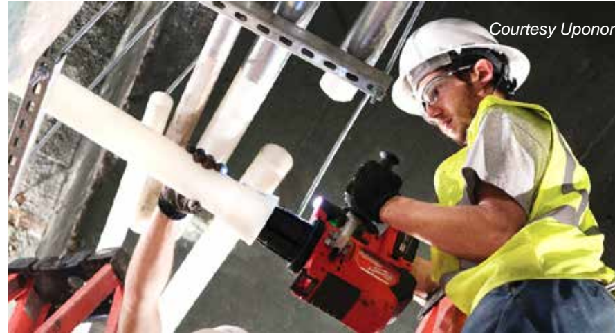
Cold-expansion PEX fitting per ASTM F1960
